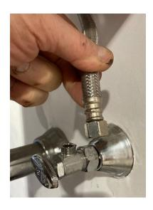
Attach the nut on the hose to this valve, and tighten gently with a wrench.
